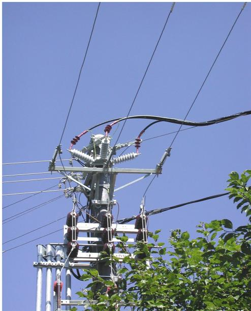
**Fig. 11.** Construction of an energy HV distribution of 22 kV with electrically shielded conductors.
