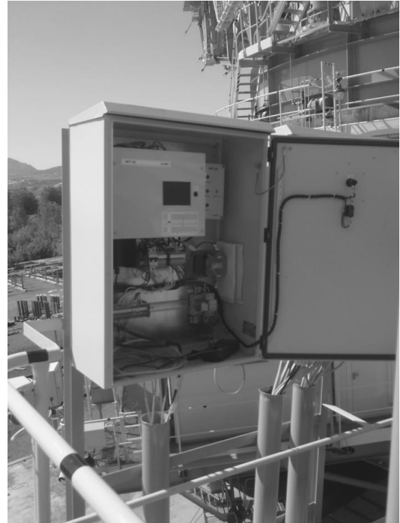
Fig. 7. HFT system installed on the KK1300 excavator, SD Bílina
